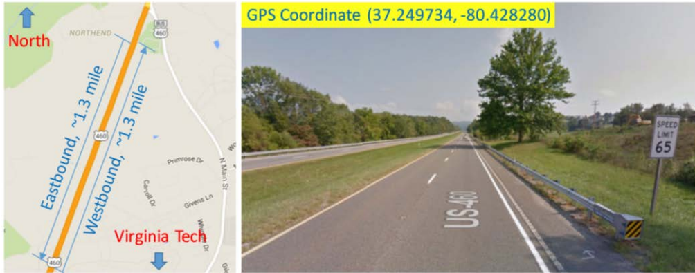
Dense graded hot mix asphalt (HMA)
